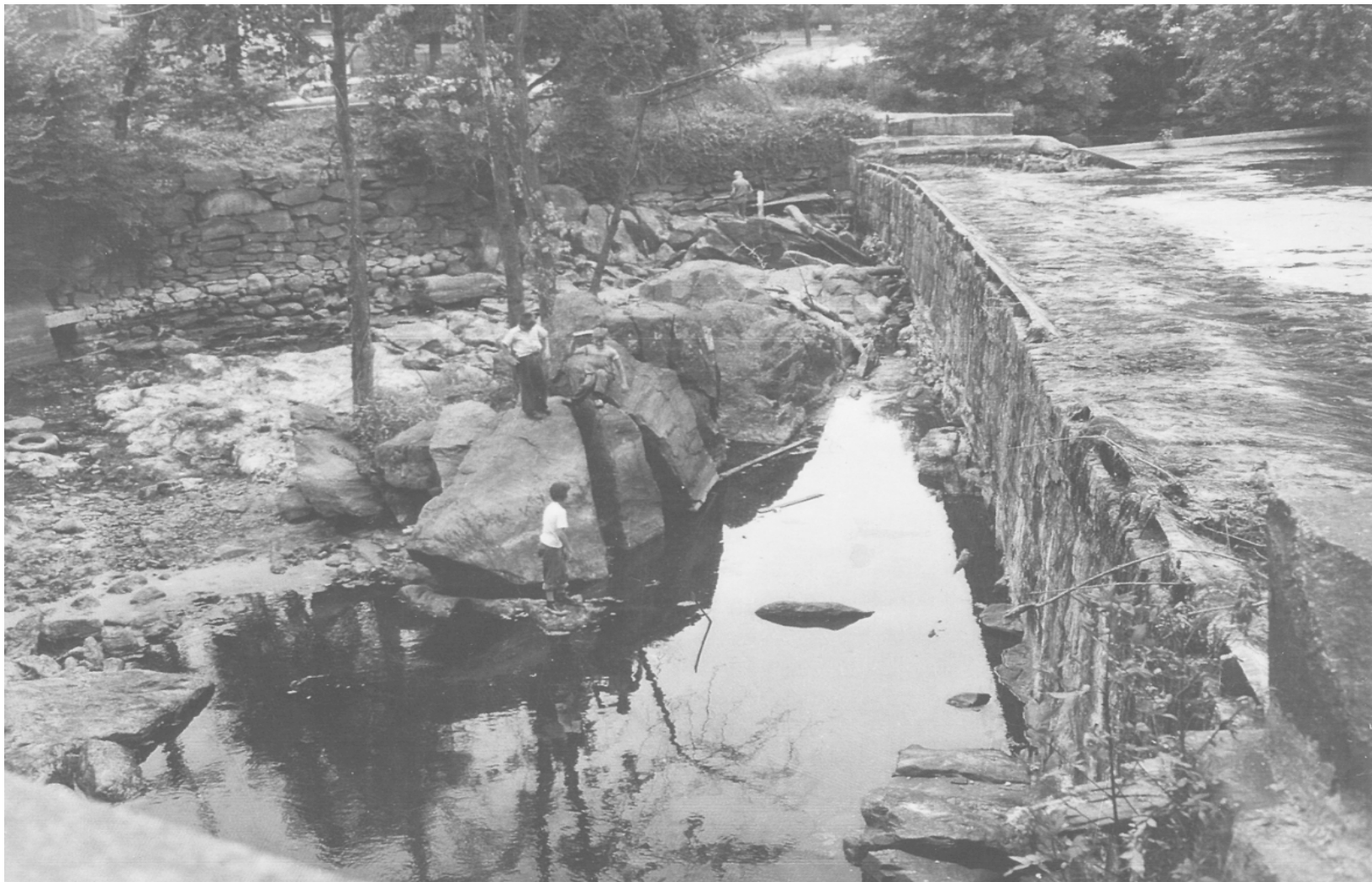
Talbot/Billerica Falls Dam, built 1828, 5.8 to 8.28' high plus 7¾" flashboards. 1957 photo
