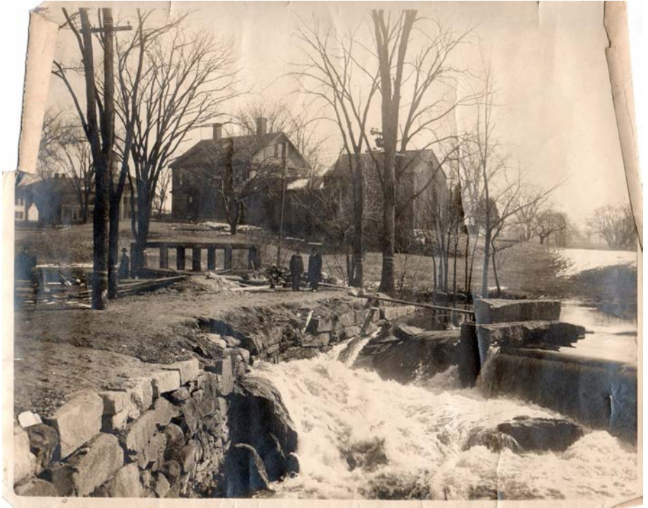
Picture showing the fishway in the Talbot Mills Dam. (Circa 1900).
