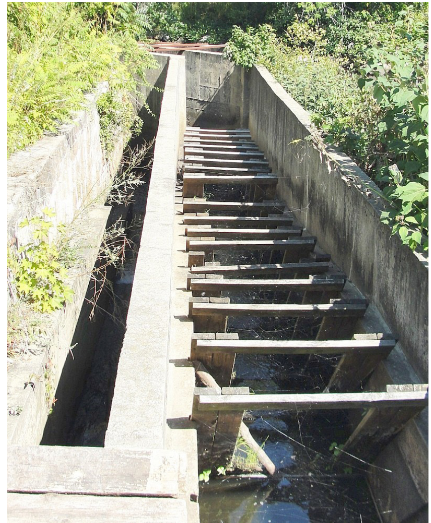
Centennial Dam bypass on left. Denil fishway for fish migrating upriver on right.
