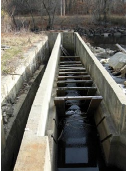
Photo D, Wamesit Falls/ Centennial Dam fishway and downstream passage
