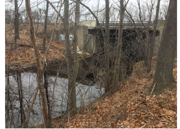
River Meadow Brook, Bridge Needed to NW
