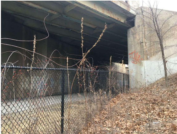
BFRT Tunnel from 495E Right of Way to NW
