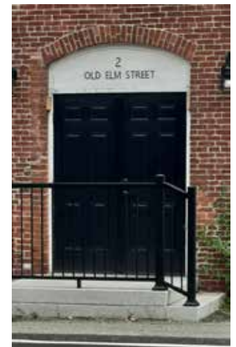
The entrance facing Old Elm Street with new metal signage above the door.
