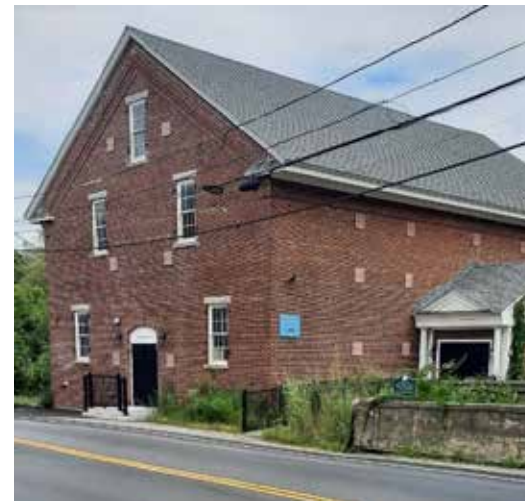
In this photo the signs are in place but the area around the building had not been cleaned-up.
