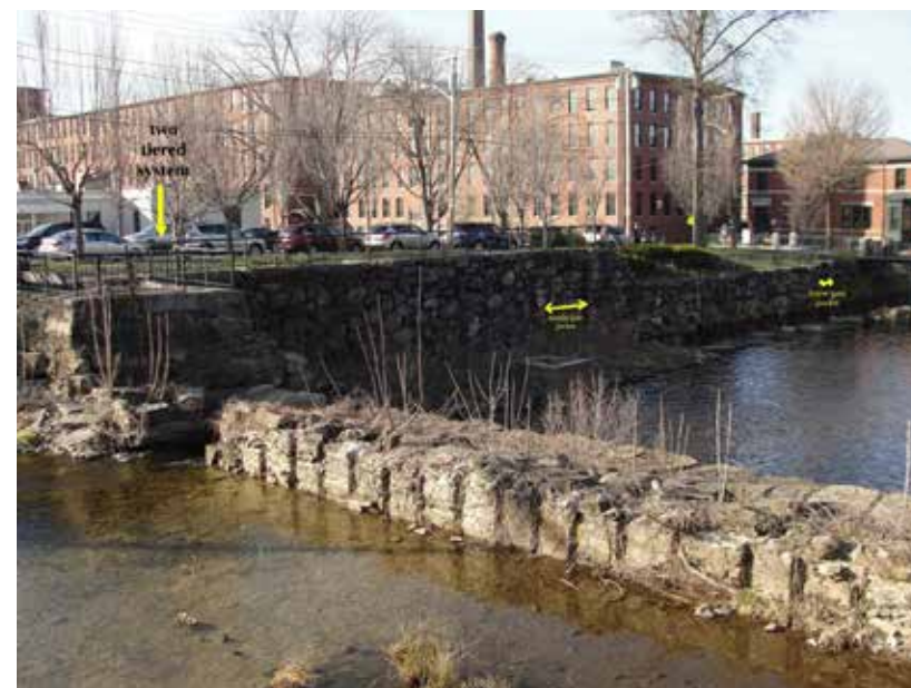
Locks with middle and lower gate pockets labeled.
