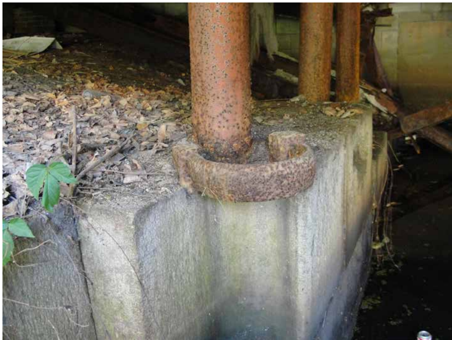
Hollow quoin and heel post collar, 11" diameter.
